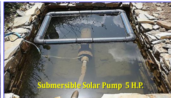
Pre Fabricated Geo Membrane Water Harvesting Tank Capacity 20000 Lit.
